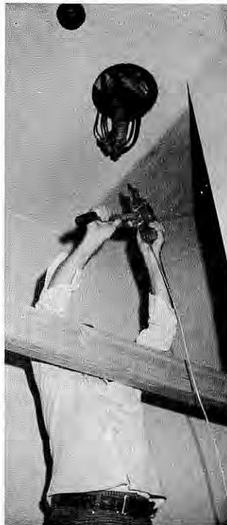
A COMEALONG was rigged to 2 by 6 timbers on landing below chamber and attached to chains lashed around blower. Here muscle power is uniting Comealong and steel cable.
