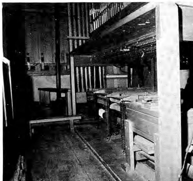
COMPACT—view shows regulators and tremulant for Vox Humana look-in through chamber door. Swell shade opening onto balcony seen in background and offsets for Flute and Diapason were aligned along the wall to left.
