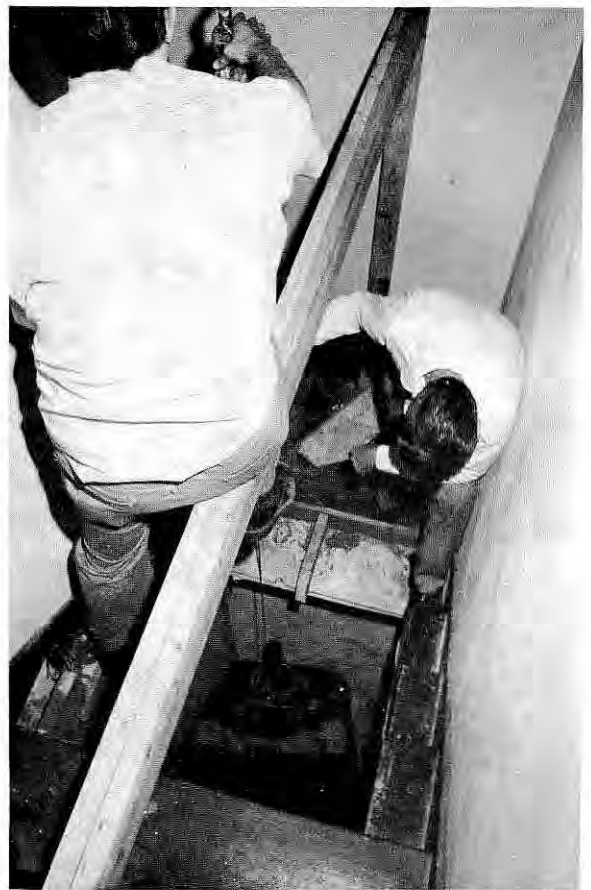
A COMEALONG was rigged to 2 by 6 timbers on landing below chamber and attached to chains lashed around blower. Here muscle power is uniting Comealong and steel cable.
