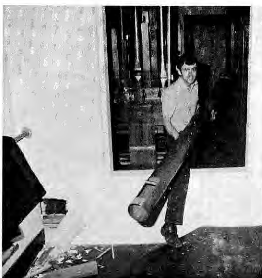
LEO MALBERG removes 8 ft. Diapason pipe through swell shade opening. Hole in wall in lower left corner was knocked into chamber to run computer lines through chamber.
